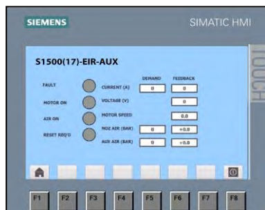
HMI screen specifically designed to monitor values
